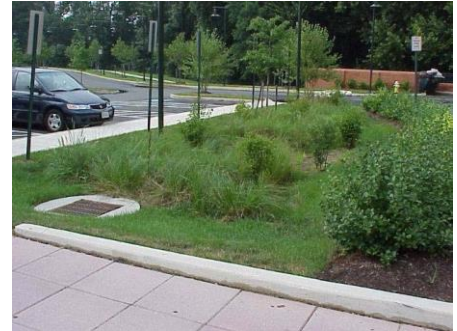
Positive Overflow: Inlet
