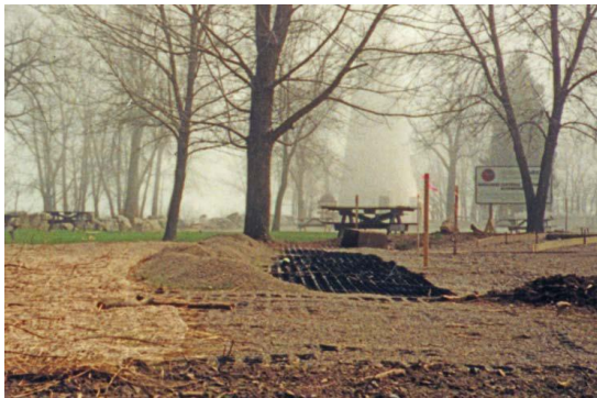
Pervious Paver Installation
