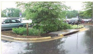
Curbed Parking Lot Perimeter Bioretention
