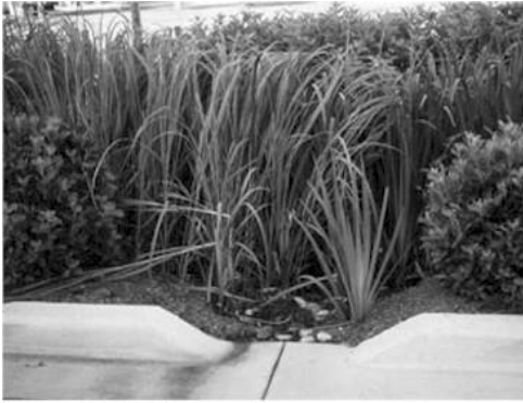
Flow Entrance: Curbs and Curb Cuts
